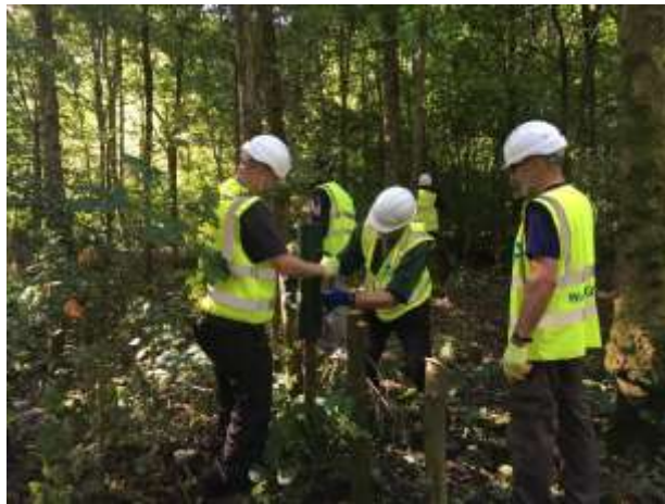
Fig 8. Volunteers installing Leaky Dams at Low Hall Local Nature Reserve
